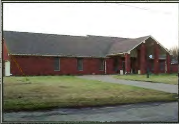
Unarticulated Residential. This residential structure appears to be significant in size. However, the straight and unbroken surfaces of the roof and exterior walls are plain and uninteresting. They add nothing to the design of the structure.
