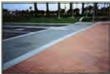
↩ Special Paving Treatment should be used at locations for emphasis, such as a corner crosswalks or at locations where pedestrian paths and trails cross local roadways. Variation of different styles can add to the aesthetic quality of the site.
