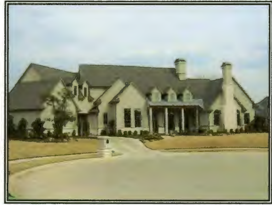
Articulated Residential. Real visual interest is created by the varied planes and surfaces of the design. Notice a variety of breaks in the roofline as well as the addition of dormers to add interest to the roof. The exterior walls have a variety of angles and offsets to add to the articulation of the structure.
