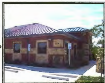
↳ Accents provided by varying the stone material and pattern add to the diversity of the structure. Accents around the windows and on the corners cause the eye to perceive articulated surfaces.
